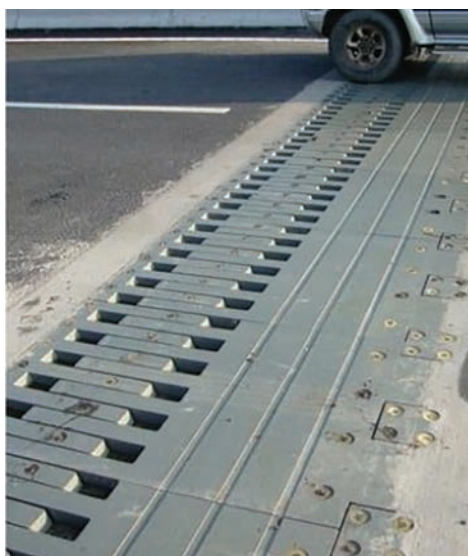
Figure 8.3 Expansion joints for safety
