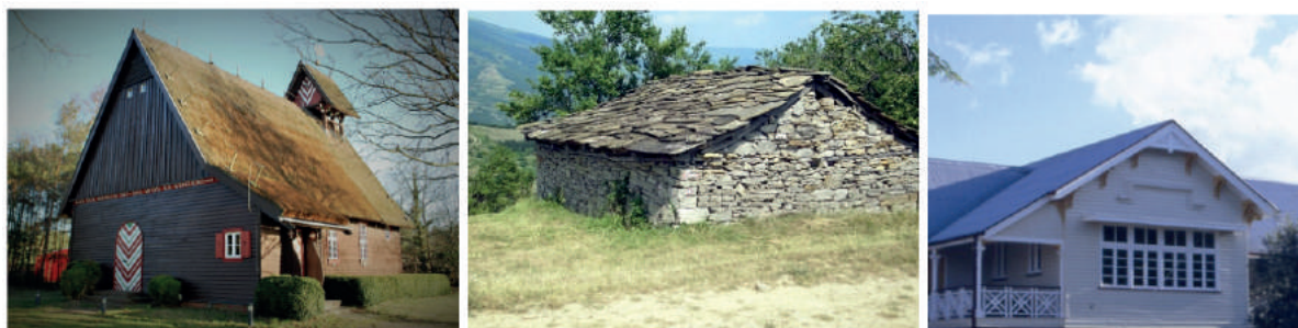
Fig. 5.3, A thatched roof, stone roof and a metalsheet roof.
