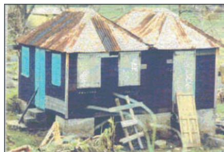
Fig 1. If natural elevation is not available construction on stilts or on artificially raised earth mounds
