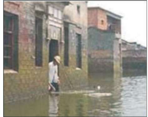
Flood disrupting normal life
