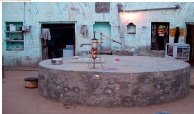
Figure 2.30: Small cylindrical underground well (tanka)
