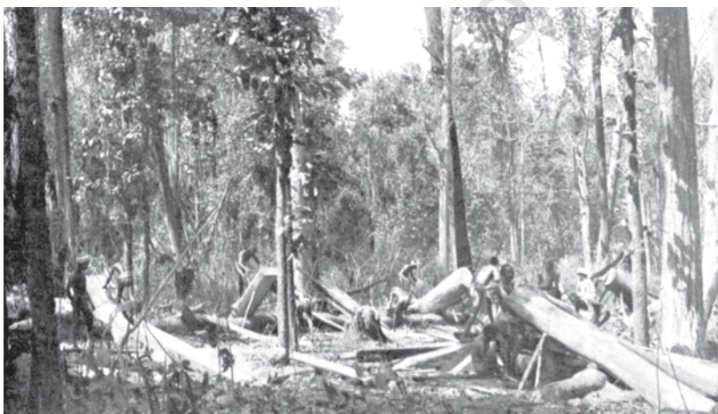
Fig.3 – Converting sal logs into sleepers in the Singhbhum forests, Chhotanagpur, May 1897.
