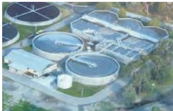
Figure 10.7 An aerial view of a sewage plant
