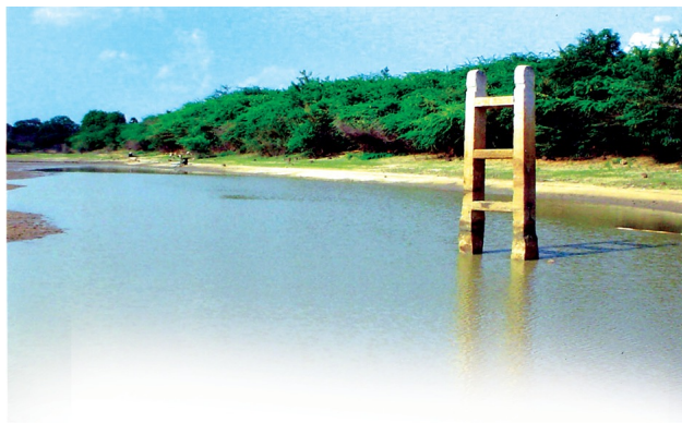
Fig 11.5 A ninth century sluice gate in Tamil Nadu. It regulated the outflow of water from a tank into the channels that irrigated the fields
