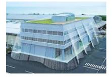
It is the building which is designed by the Japan which is strong enough to face the wild earthquake. The strings are being attached by the fibre.
