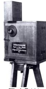
Fig1.7 (A) Cinematographe in camera mode
