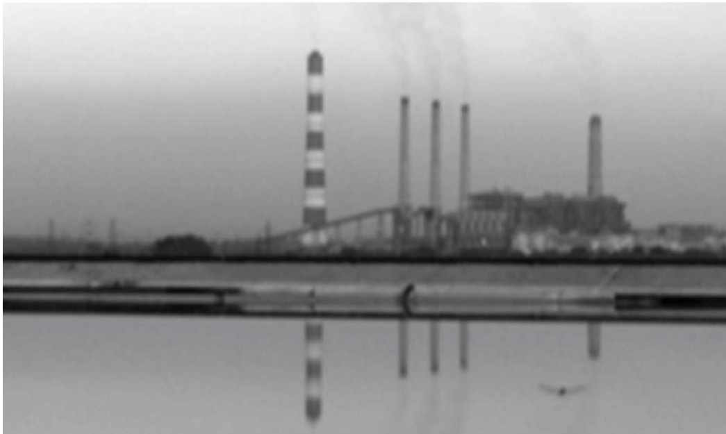
Infrastructure : Power Generation
