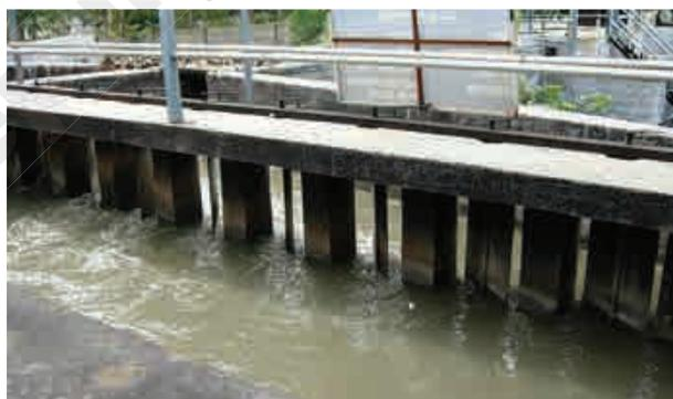
**Fig. 18.4** Grit and sand removal tank
