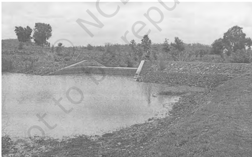
A small dam
