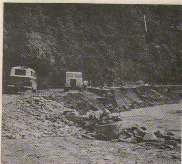
4.C A landslide after flood has damaged the road Jabatai Penerangan Malaysia
