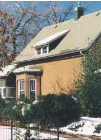
Energy is conducted from the inside to the exterior more rapidly on the part of the roof where the snow has melted. The dormer appears to have been added and insulated. The main roof does not appear to be well insulated.
