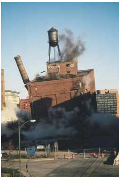
Figure P10.51 A building demolition site in Baltimore, MD. At the left is a chimney, mostly concealed by the building, that has broken apart on its way down. Compare with Figure 10.19. (Jerry Wachter/Photo Researchers, Inc.)
