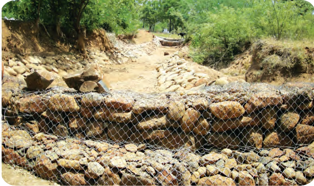
Fig. 6.12 : Gabion dam on stream
