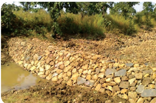
Fig. 6.11 : Loose rock check dam
