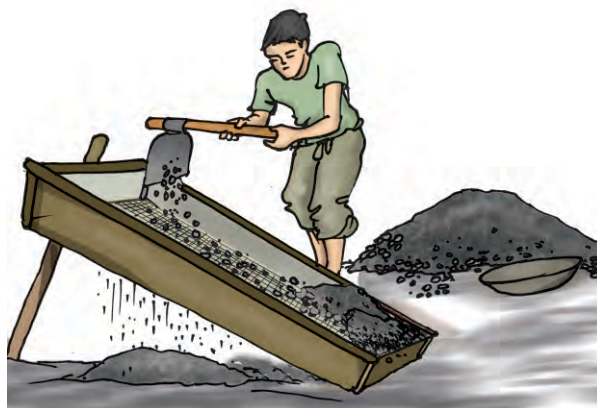
Fig. 5.7 Pebbles and stones are removed from sand by sieving
