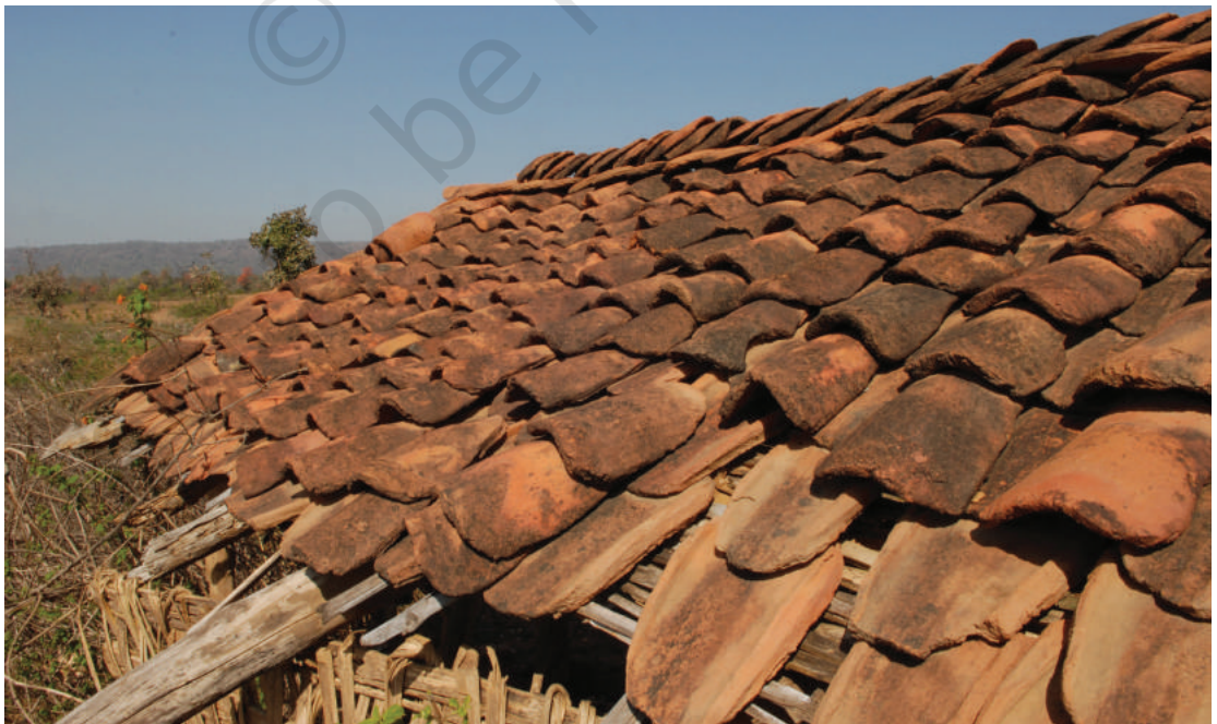
Clay roof-tiles, Madhya Pradesh
